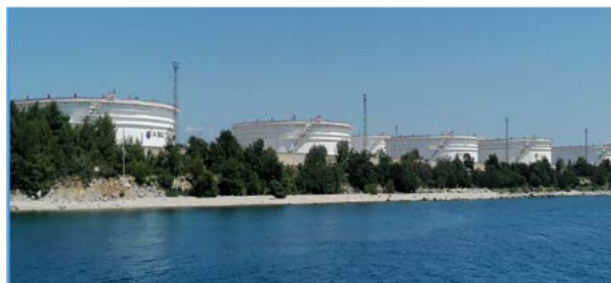
Figure 3: Five of the twenty oil tanks owned by Janaf, the Croatian national oil company (Photo by the author).
