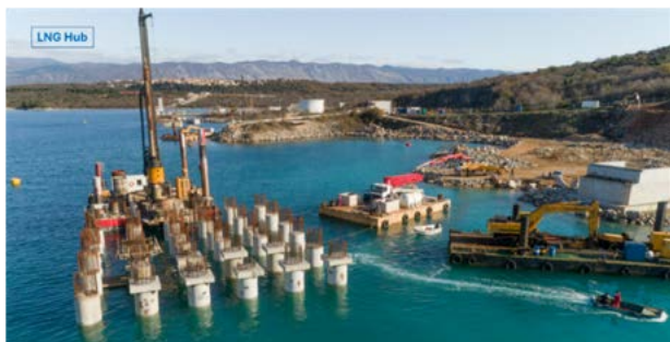
Figure 4: The construction of the docking facility for the LNG-Hrvatska, in 2019-2020. In the background, on the hills, the village of Omisalj (Photo by Balkan Insight).
